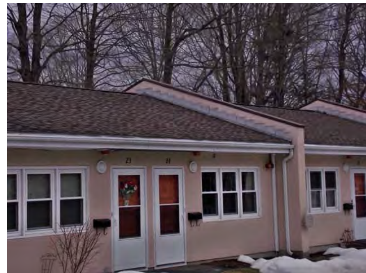
The roofs are covered with architectural shingles and unit entry doors are protected with storm doors.
