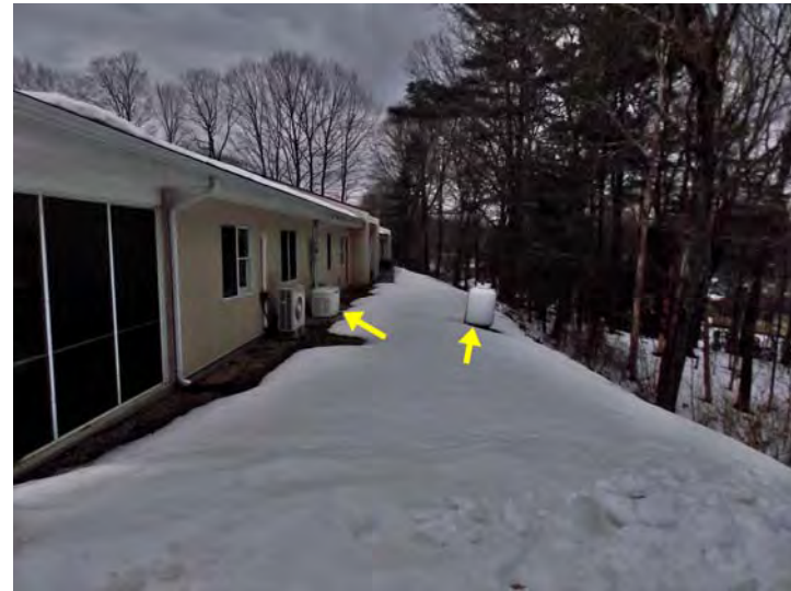
The emergency generator (left) uses propane (storage tank on right) to provide emergency power to the community room.
