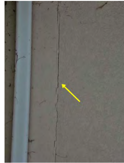
A close-up of a caulked control joint that has cracked.
