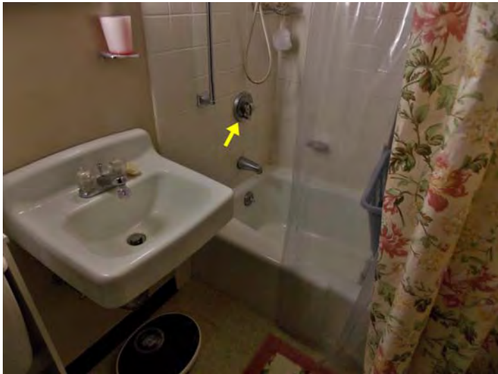
Most bathrooms have wall-hung sinks and tubs with an anti-scald mixing valve.
